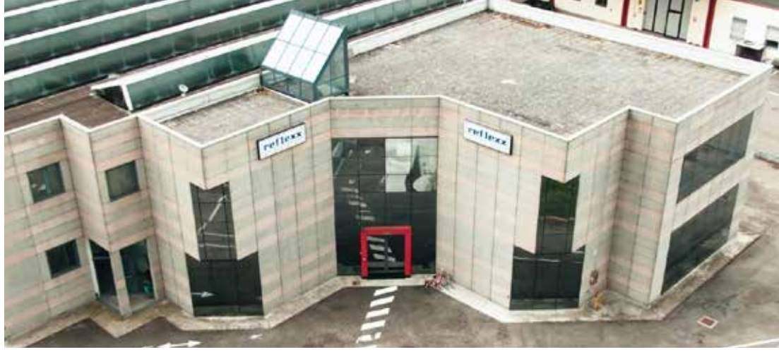
● HEADQUARTER Viadana (MN)
